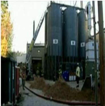
*A massive fire and explosion in the dust collection system of a New Hampshire wood pellet manufacturer demonstrates the need for adequate system design to prevent combustible dust explosions in general industry.*
